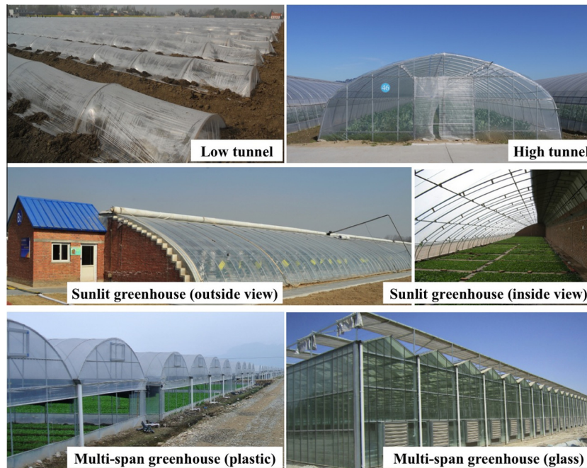
Fig. 1. The greenhouse structures adopted for vegetable production. Low tunnels (plastic row cover), high tunnels (walk-in tunnels), sunlit greenhouse (Chinese solar greenhouse) and multi-span greenhouse (plastic and glass covered).
